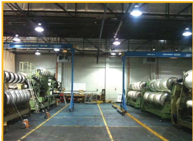
The two gantries at the start of their 35m path.
