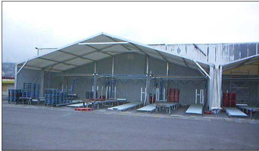
Installation on site
